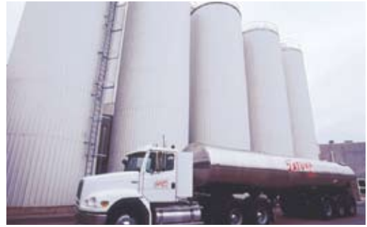
Silos for storage of raw milk at a processing factory
