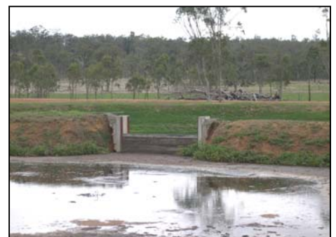
Settling basin with drop board weir
