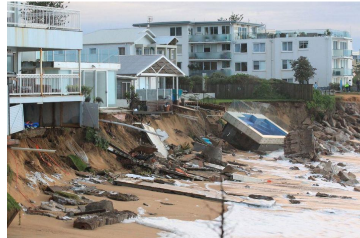
Storm surge, Sydney 2015
