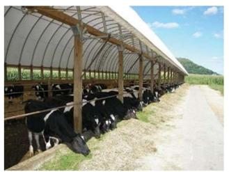
Figure 8. Composting barn with external feed-bunk and curtain. Source; https://www.pinterest.com.au/pin/650277633668970825/
