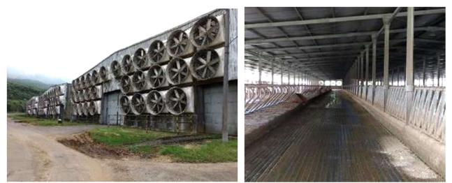
Figure 23. Tunnel free-stall dairy barns with extraction fans and clear plastic walls (Source P Chamberlain, Indonesia)
