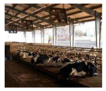
Figure 21. High Volume Low Speed fans in a free-stall barn with open sides (Source P Chamberlain, India)
