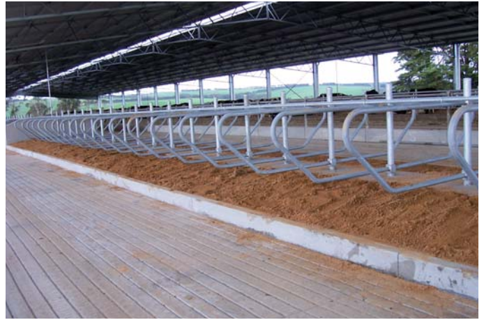
Figure 7.4 – 4-Row Covered Freestall with sand bedding, central drive alley and 2 cow alleys
