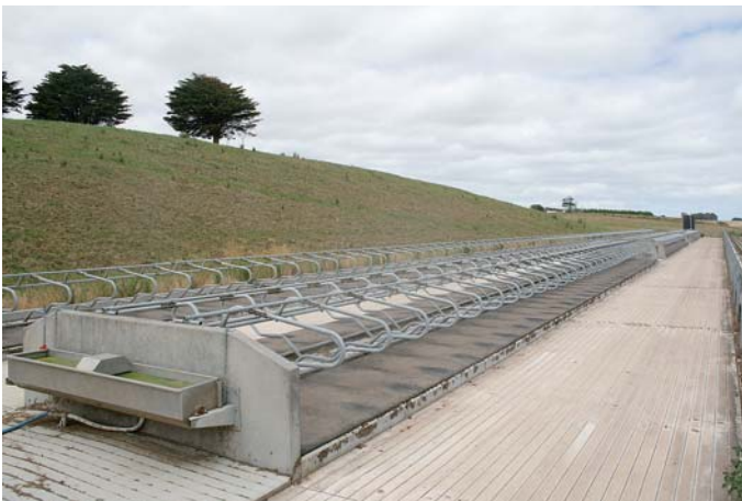
Figure 7.5 – 6-Row Uncovered Freestall with rubber matting, central drive alley, 2 feed alleys and 2 cow alleys
