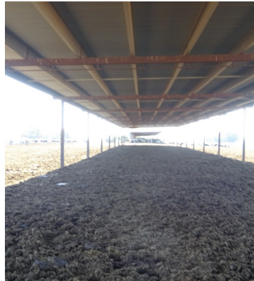
Low roofed drylot bedding pack shelter
