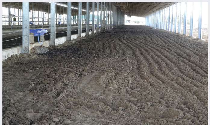
Double bedding pack shelter with covered feed lane that has a sand bedding pack (non-composting)
