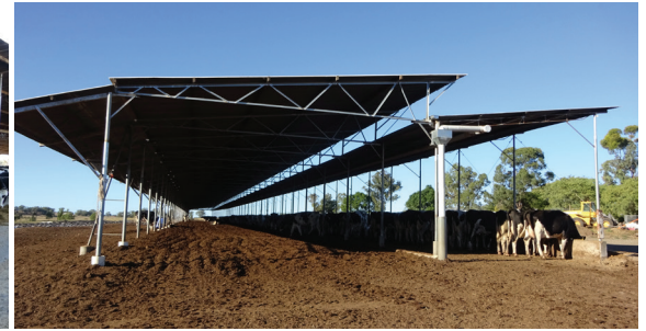
Single bay compost shelter with uncovered feeding area
