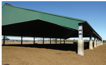
High roofed drylot bedding pack shelter and associated
