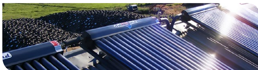
Image: Example of evacuated tube hot water system on a dairy farm.
