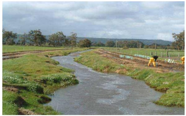
Drain streamlined and fenced to turn the drain into a functioning stream and prevent stock from having access to the watercourse.
