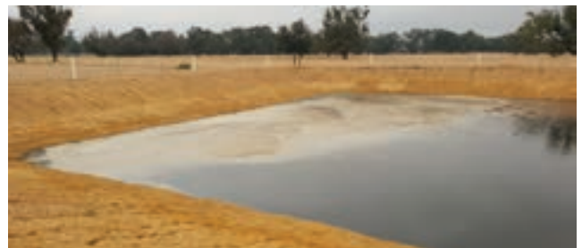
Upgraded effluent pond, Harvey
